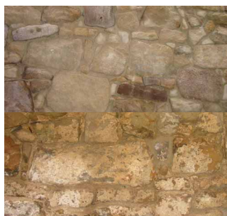
Surface cleaning - before and after
