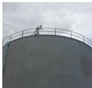
Fuel tank coating removal
