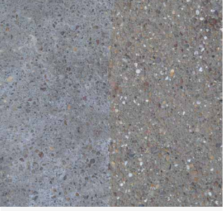
Floor tile adhesive removal - before and after
