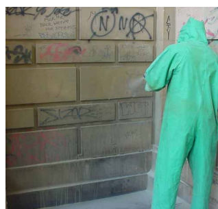
Sand stone cleaning
