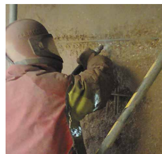
Concrete cutting
