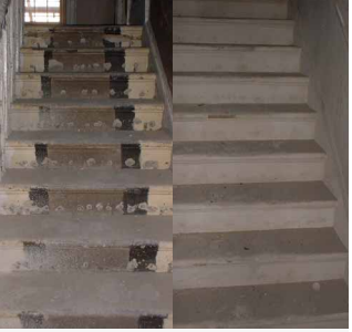
Grade II listed building stone steps - before and after
