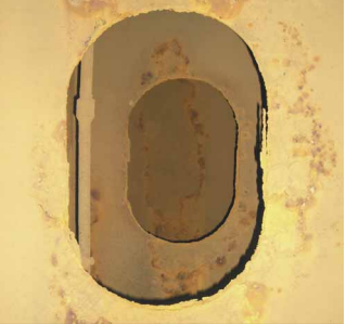
Ballast tank maintenance
