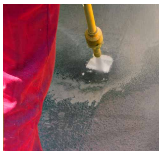
Highway line removal
