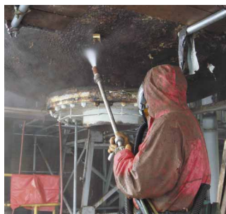
Asbestos limpet residue removal
