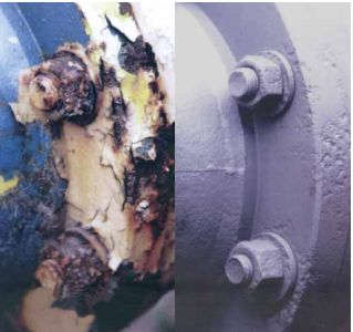
Flange maintenance - before and after
